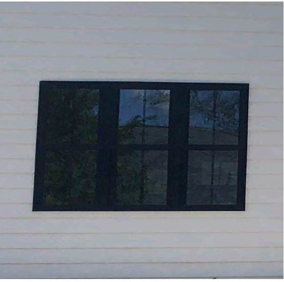
FIBER CEMENT BOARD & BATTEN / LAP SIDING
