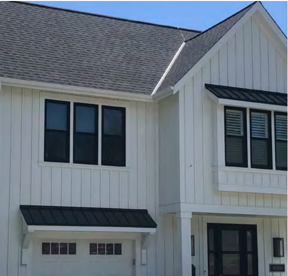
ASPHALT ROOFING WITH METAL ROOF ACCENTS
