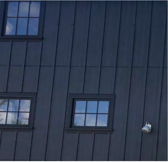
FIBER CEMENT BOARD & BATTEN SIDING
